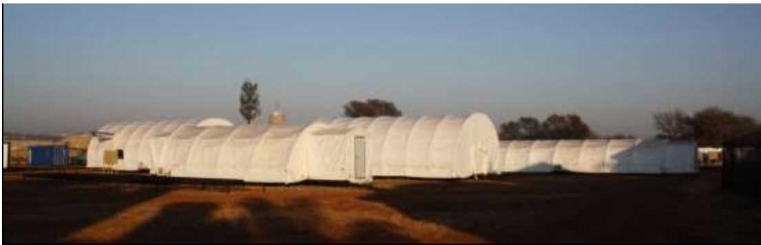
Fig 1: General view of part of the 50-man Camp
