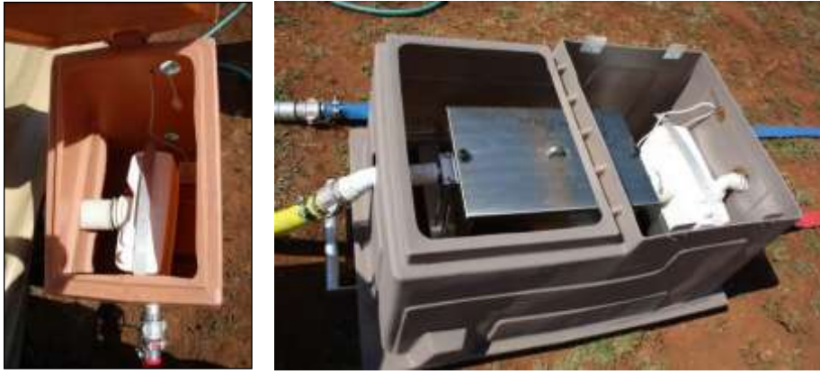
Fig 18: Macerator pump (left) and the integrated fat trap and macerator pump unit (right)
