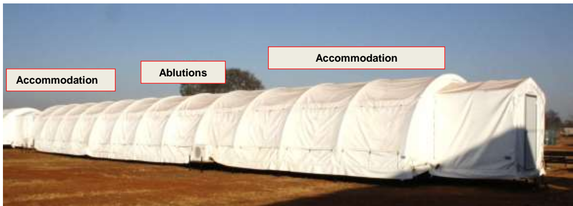
Fig 3: A Warrior based accommodation block consisting of three 4.8m x 9.6m shelters with ablutions in the center.
