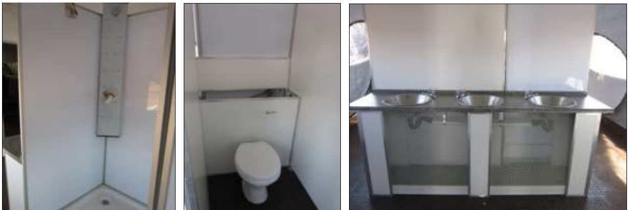
Fig 4: Ablution facilities from left to right: Shower cubicle, toilet and washbasin set.
