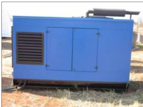
Fig 15: 150 KVA diesel generator (left) and the Synchronisation and load sharing panel (right)
